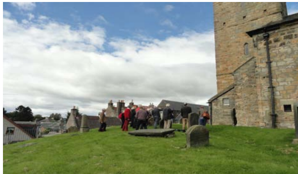
The mediaeval tower of Markinch Parish Church
